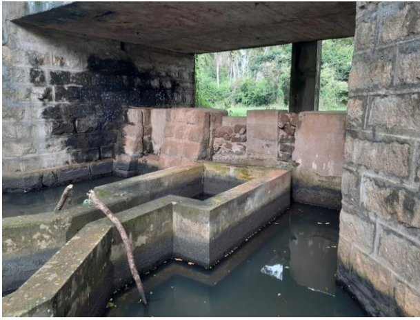
Figure 18: Ganthiriyagama Tank - Ancient Sluice Gate Repaired and Used until the 1980s
