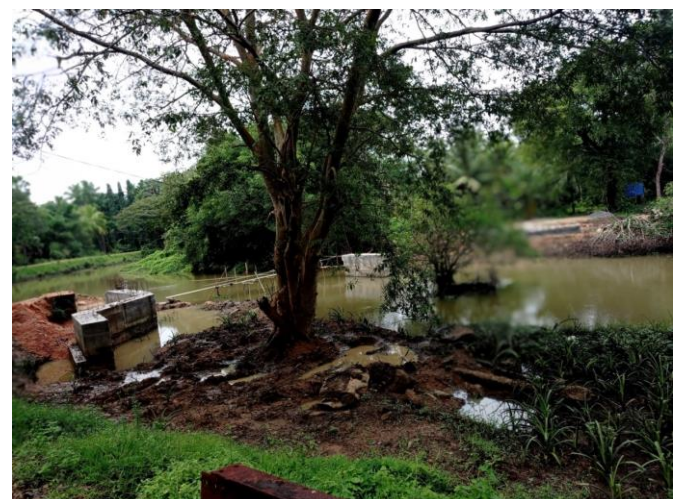
Figure 4: A new Bridge is being constructed at Amunu Gilma 3
