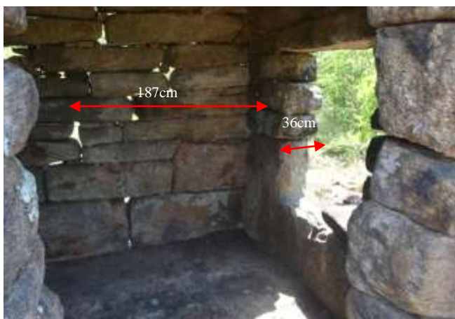
Figures 4. Inside of the building
